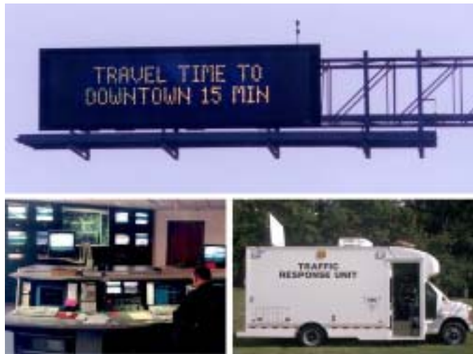
MONITOR elements include (clockwise from bottom right) service patrols, traffic operations center, and variable message signs.
